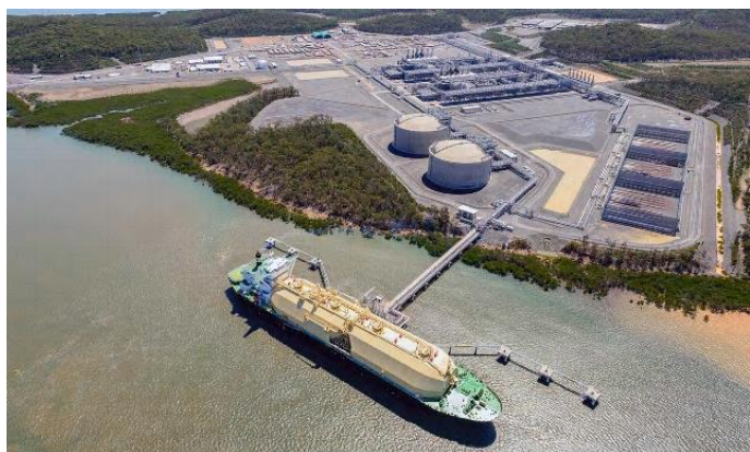
Origin Energy's Australia Pacific liquefied natural gas facility at Curtis Island in north Queensland. The Tax Justice Network says Australia is set to become the world's largest exporter of LNG by 2021
